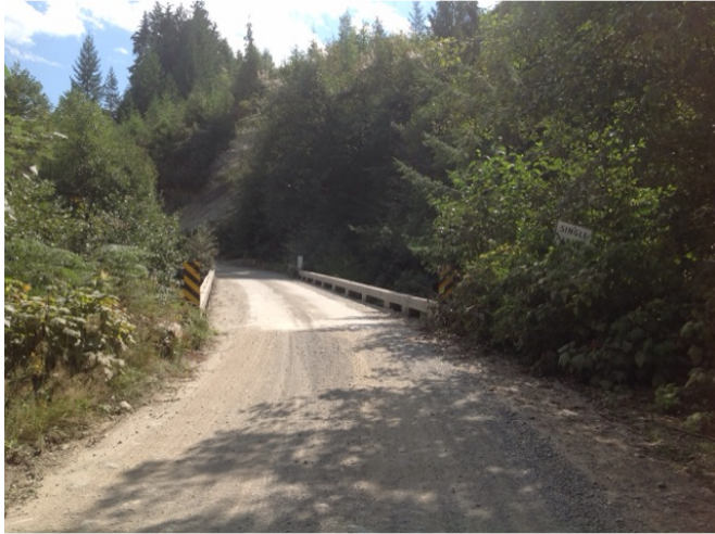
Approach from Left Bank when facing downstream
