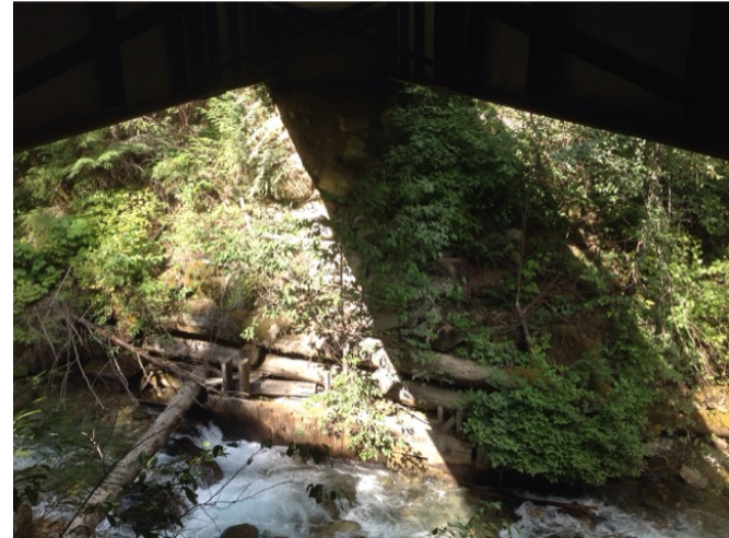
Left Bank Abutment when facing downstream
